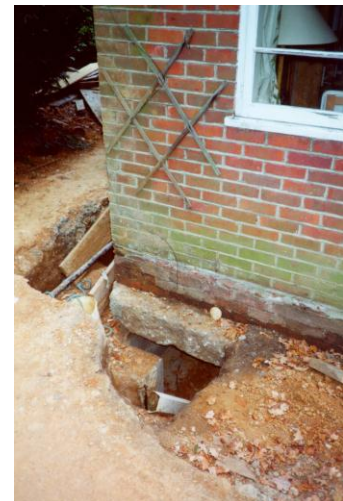
Figure 5 - House underpinning necessitated by soil-related subsidence. ( S. Hallett )
