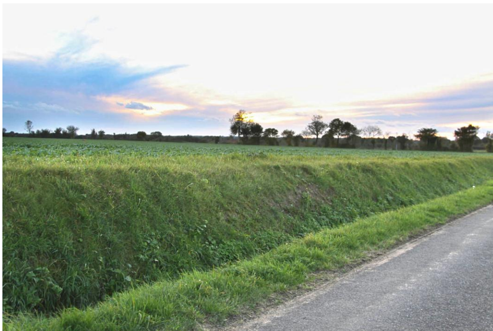
Figure 11 - Road at lower level to surrounding field due to hundreds of years of rural traffic in Suffolk (Photo: T. Farewell)
